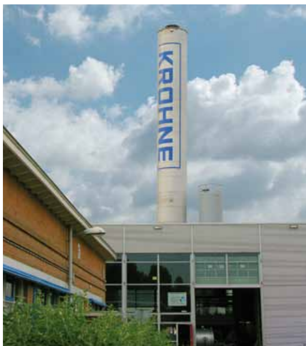
Figure 4.1: 44 meter high calibration tower at KROHNE Altometer
