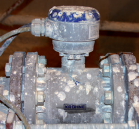
OPTIFLUX 5000: measuring tube made of oxide ceramic when used in the chemical industry
